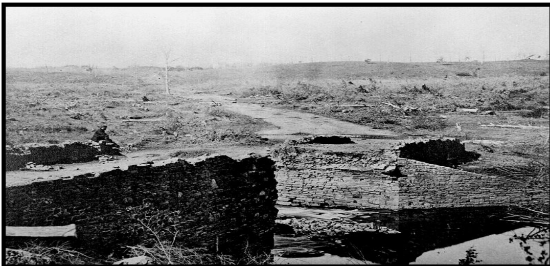
Ruins of Stone Bridge at Bull Run Creek; 2 nd Battle of Bull Run or 2 nd Manassas, March 1862, Captain Girardey Assumes a Command
