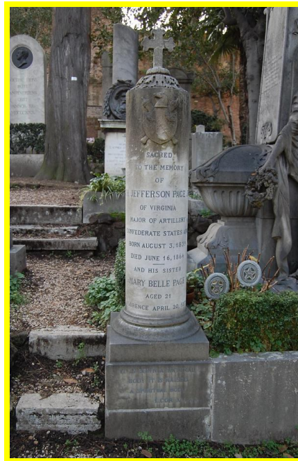
One of the memorial pylons at the tomb. This one is devoted to Thomas J. Page jr., Major of Artillery, ANV, and his wife Mary Belle. Although not so badly deteriorated, water runoff streaks can be seen on this and the other column.
