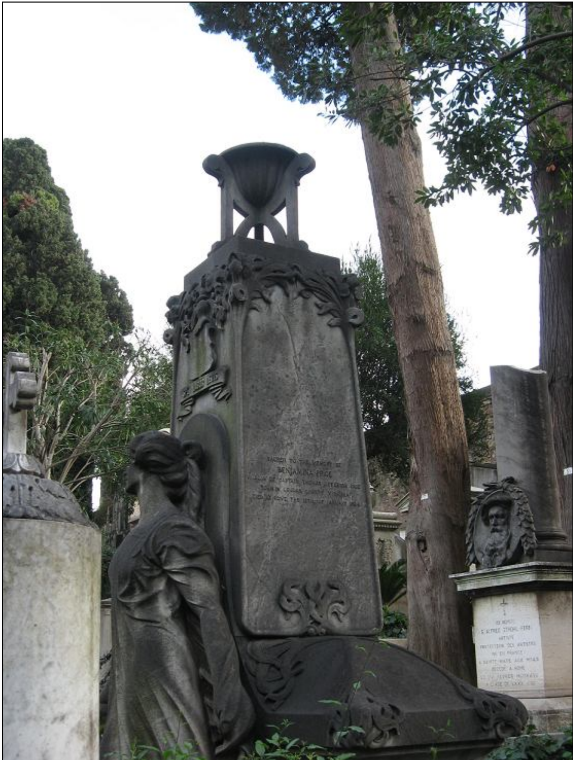
White marble, covered with the dirt of more than a century
